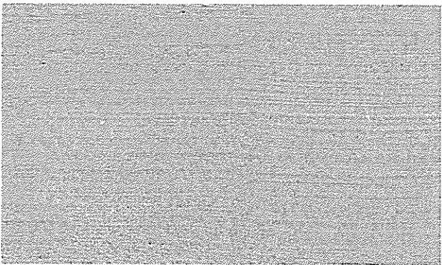
Footpath paving along James Street - concrete with broom finish
