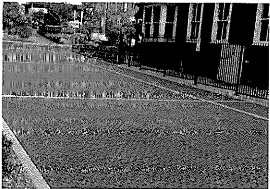
Permeable Paving - Ecotrihex with concrete banding
